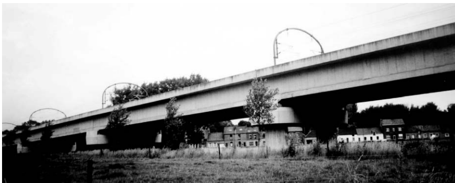
Fig. 1. View of Antoing Bridge.
